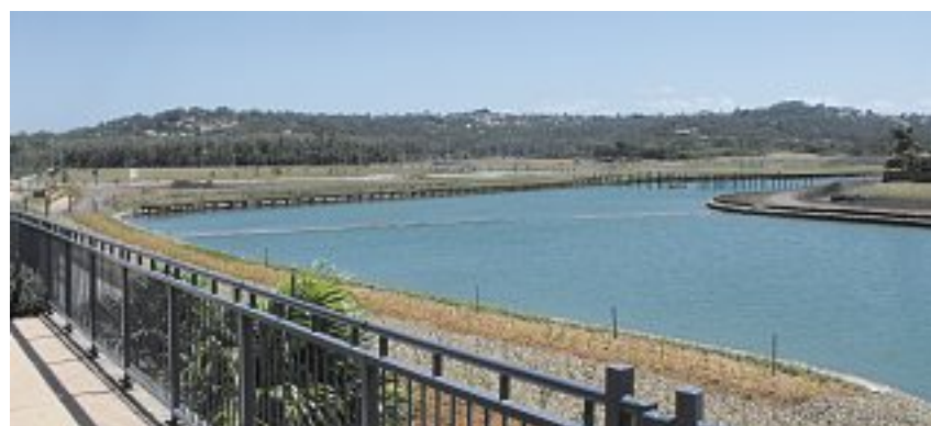
TAKING SHAPE: Work on the $800million Sunshine Cove is well under way.
